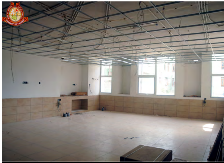
Research Labs Under Renovation
